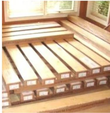
Cartons elevated from subfloor and cross stacked for air circulation
